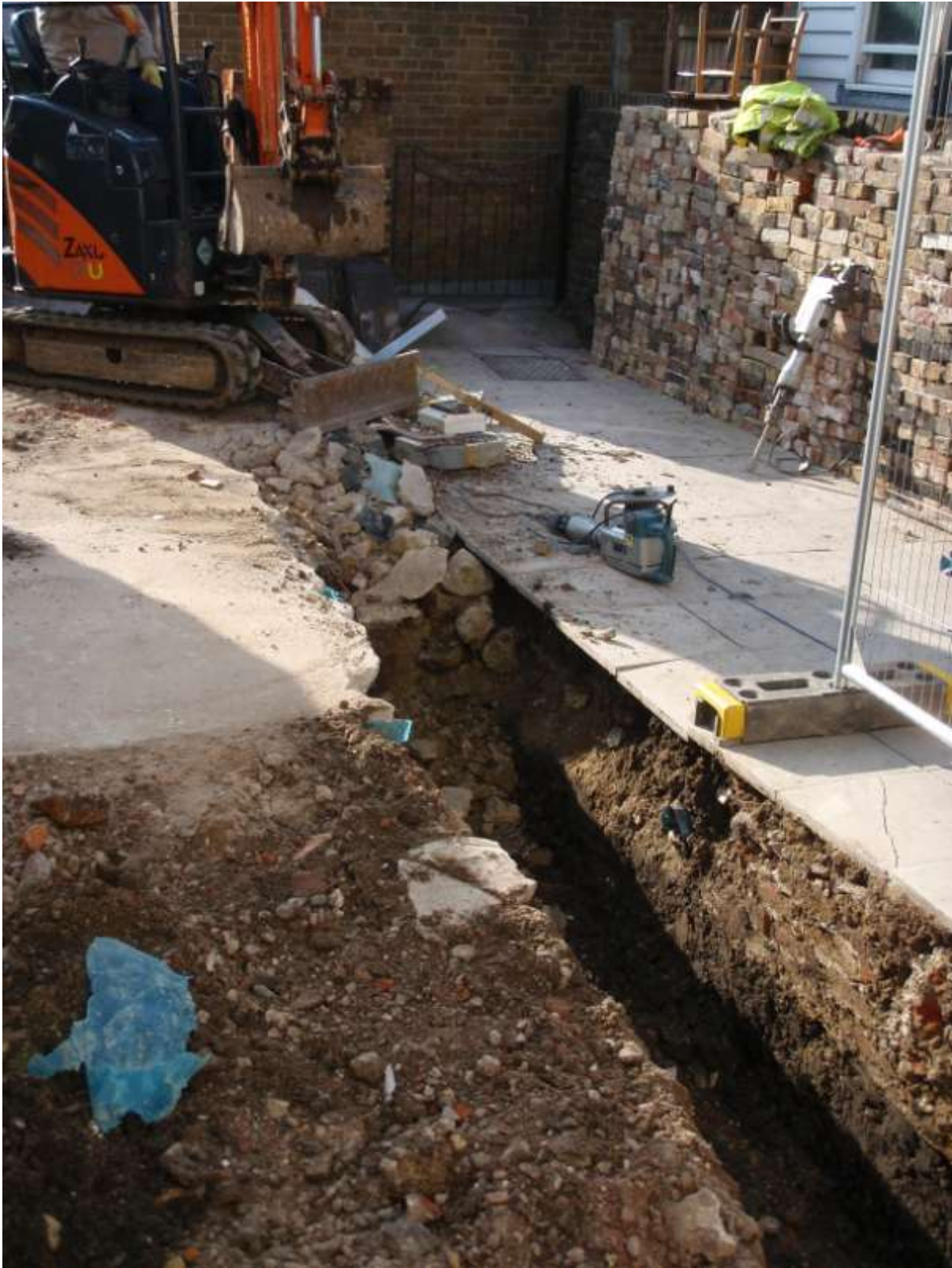
Plate 3. View showing digging of foundations
