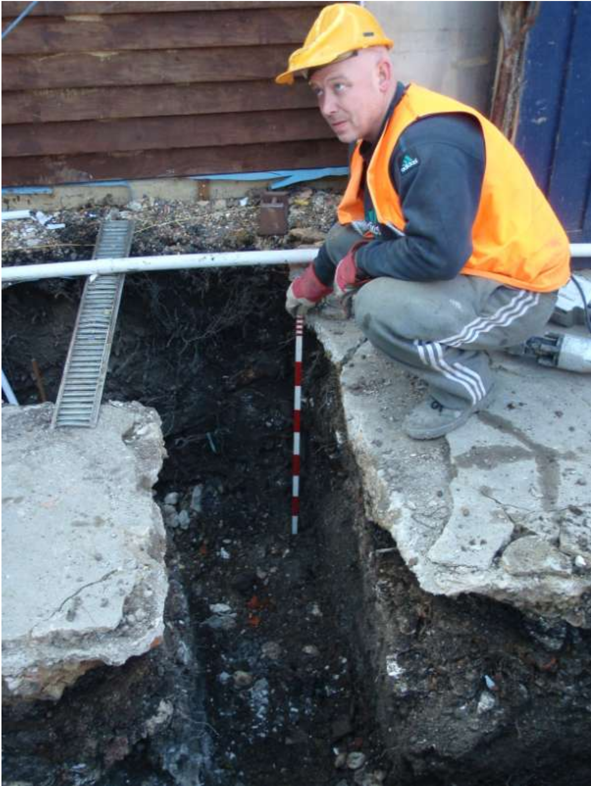
Plate 4. The site showing cutting of foundation trenches
